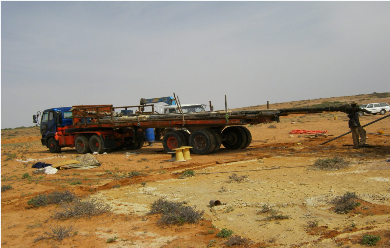
FLAT TRAILER OR HEAVY DUTY TRUCK carrying all equipment
